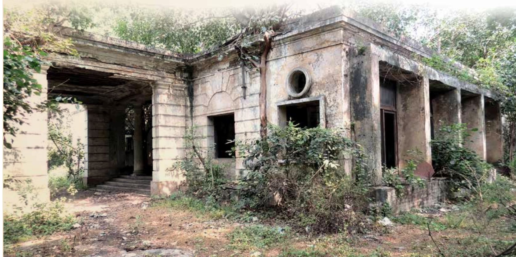
15 Rajpur Road as it exists now
